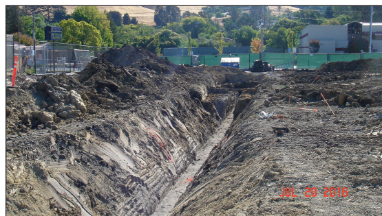
Storm water and sewer drain piping trench
